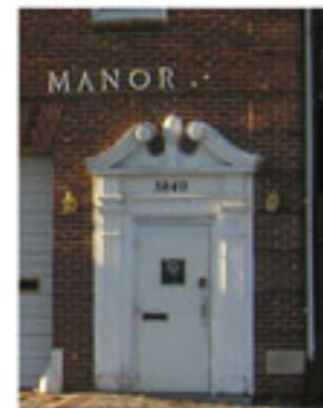
BUILDING FACADE-- RED BRICK
