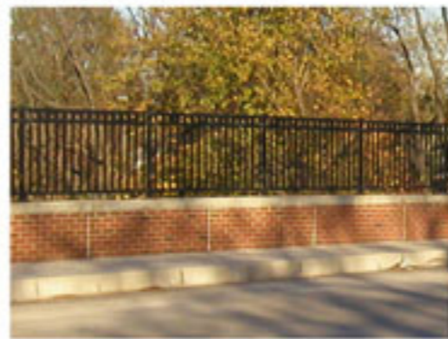
BRIDGE WITH RAILING
